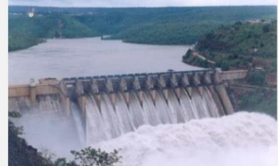
Srisailem Dam, Mahabubnagar/Kurnool
