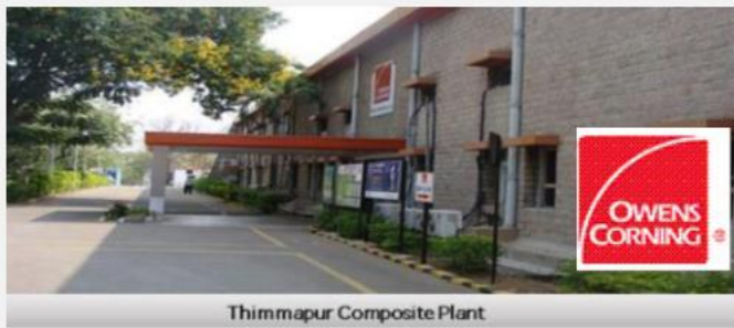
Thimmapur Composite Plant
