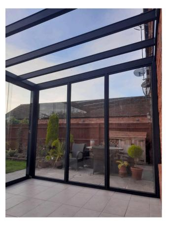
Pigato Glass Roof with fixed glass side and front sliding glass doors.
