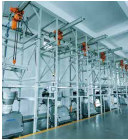
原料改性车间 Compostable Material Modifying Workshop
