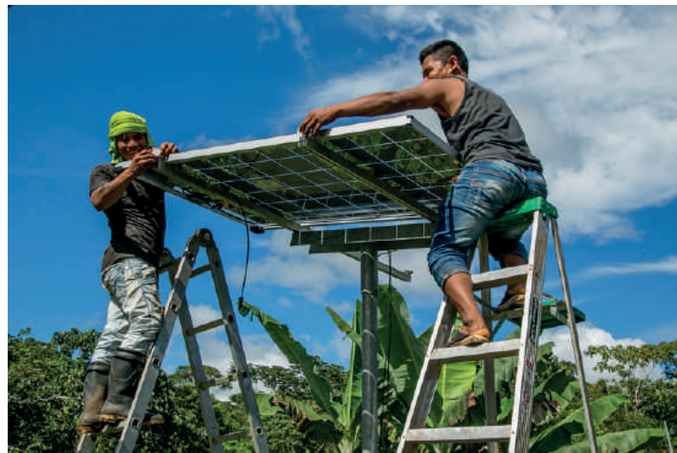
Solar home system installation in the community of Mañoko in the Peruvian Amazon
