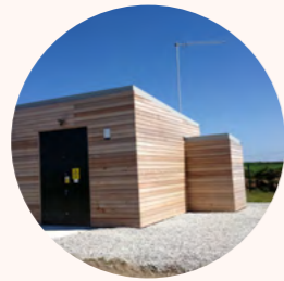
Substation Holds the switchgear and is the electrical exit of the site.
