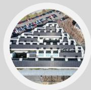
Trust's Heelis HQ solar system, expanding it from 60kWp to 344kWp with a sustainable, behind-themeter design using recycled components.
