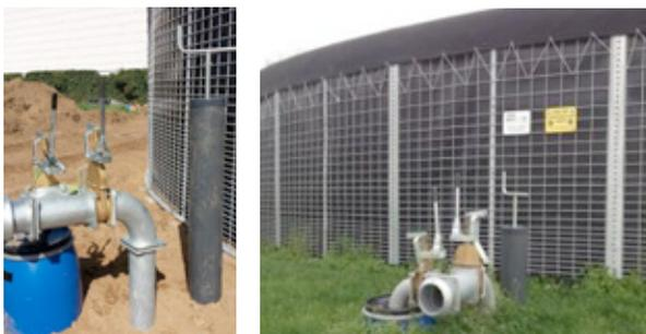
Netsilo systems are suitable for storage of all liquid volumes from 192m<sup>3</sup> to 1382m<sup>3</sup>. These liquids can be stored with optional floating cover. A concrete base is not required allowing for a quick installation and is easily movable to another site. The discharge station is used for filling and emptying the above ground tank and conforms to SAFFO requirements.
