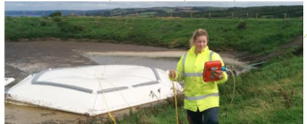
LagoonQUBE is a flexible, removable lagoon cover that operates as an anaerobic digester. It is designed to float on top of a lagoon or open top tank to collect biogas and harvest rain water.
