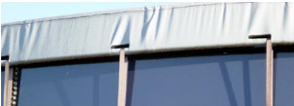
The AMTC tensioned cover is the ideal solution for your above-ground circular tank. The roof can be placed on almost any type of silo, e.g. steel or concrete. The materials used are ideally suited for manure storage systems.
