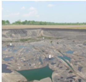
A floating cover is a practical alternative to a roof on an above-ground circular tank or lagoon. Available in sizes from 9 – 35m diameter, and bespoke design for lagoons these covers are customised for clients and fitted to Dutch BRM standard for slurry storage.
