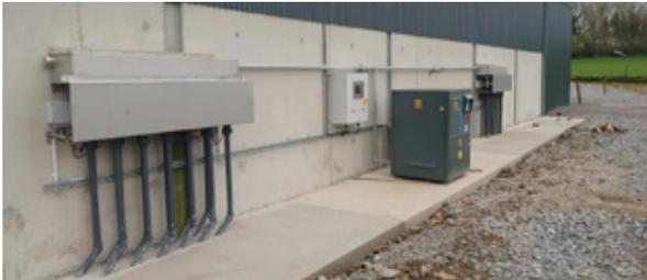
Automatic Slurry Bubble System (ASBS) is a cost-effective, energy efficient method for improved quality in slurry storage. The bespoke aeration system blows air through relay valves and circuits fixed to the tank base.
