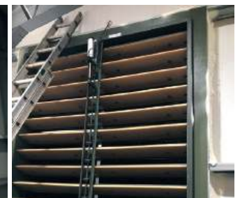
LOUVRE LIGHT FILTER FITTED
