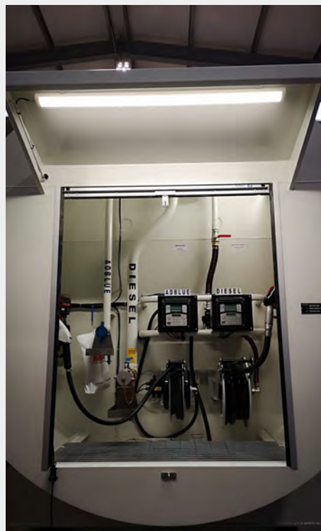
FULL-HEIGHT CABINET HOUSING DUAL DISPENSING SYSTEMS FOR BOTH DIESEL AND ADBLUE
