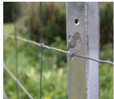
Step 5 Push the wire down, the keeper will automatically close
