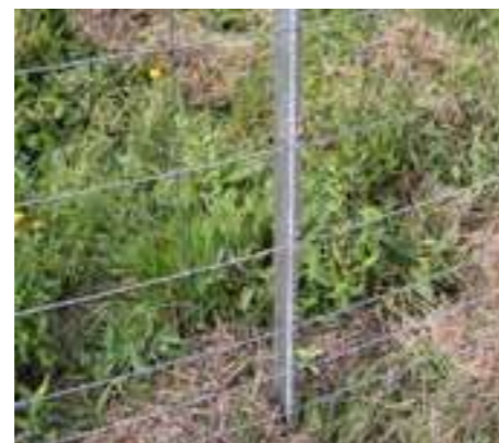
Step 3 Place Clipex® posts between vertical wires at even spacings then drive in
