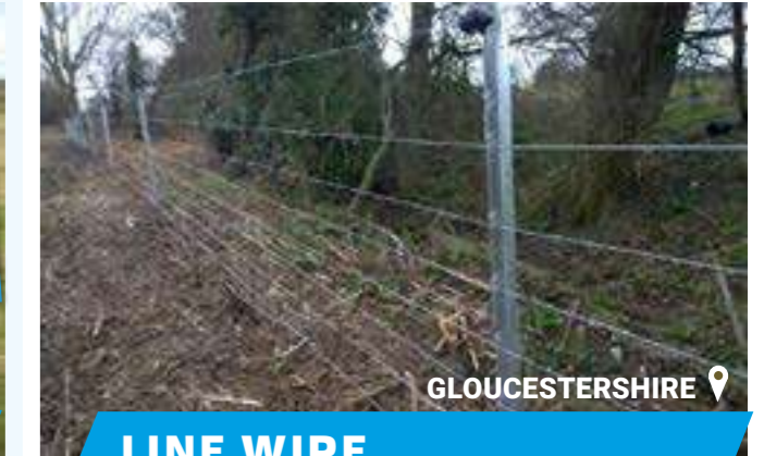
LINE WIRE FLOOD FENCE
