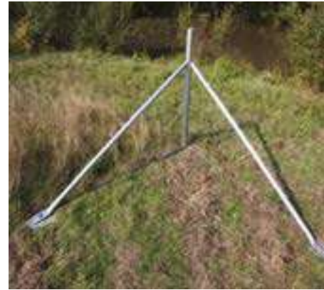
Step 1 Secure your corner/end strainer
