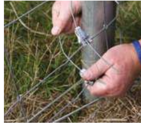
Step 2 Tie off wire netting both ends and tension to middle until upright and taut
