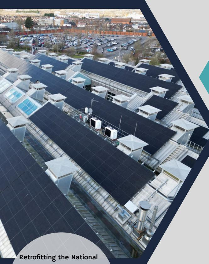
Retrofitting the National Trust's Heelis HQ solar system, expanding it from 60kWp to 344kWp with a sustainable, behind-the-meter design using recycled components.
