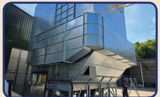
Optional Furnace Mesh Enclosure, for use in dirty environments where there is a lot of chaff to prevent accidental fire.
