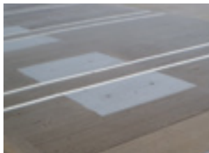
Root fixed flush to the slab
