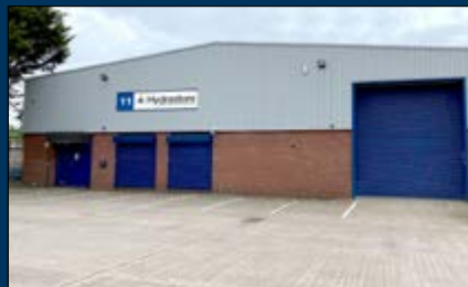
Hydrastore fluid transfer division
