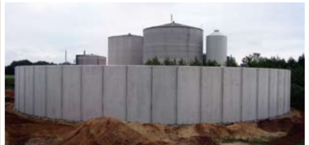
Tank installation period typically 1-2 days
