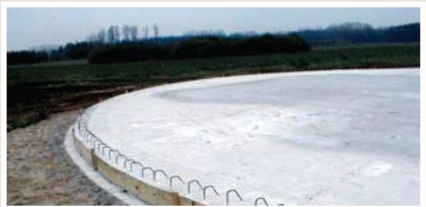
Reinforced cast in-situ concrete base
