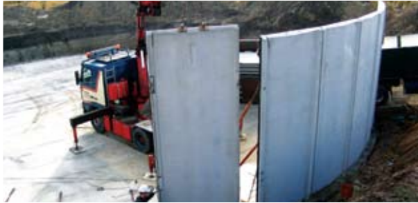
Fast track installation
