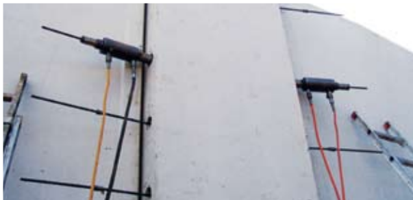
Robust Construction – internal high strength steel tendons
