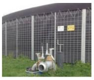
Netsilo systems are suitable for storage of all liquid volumes from  $192\text{m}^3$  to  $1382\text{m}^3$ . These liquids can be stored with optional floating cover. A concrete base is not required allowing for a quick installation and is easily movable to another site. The discharge station is used for filling and emptying the above ground tank and conforms to SAFFO requirements.
