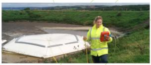
LagoonQUBE is a flexible, removable lagoon cover that operates as an anaerobic digester. It is designed to float on top of a lagoon or open top tank to collect biogas and harvest rain water.
