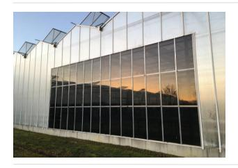
Transparent Solar PV Glass - technology deployed in greenhouses as a thermal power generating window. Offering improved and regulated environmental control (heating, lighting, irrigation, etc.) while generating clean renewable energy to automate, electrify production and reduce the operational carbon footprint.
