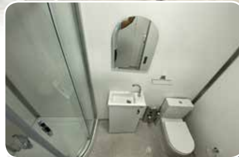
Toilet & Shower Area
