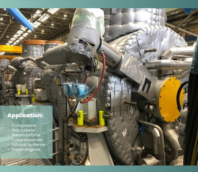
Acoustic blankets are a versatile and functional solution for noise reduction. They are a flexible insulation system, completely removable and reusable. This system is easy to install and remove on field. Acoustic blankets are tailor made on noisy machinery and they reduct noise at the source. This system is applicable in each installations, indoor or outdoor and even on many high heat equipments.
