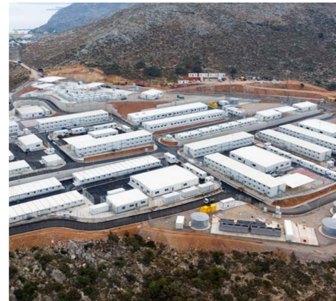
Accommodation Camps Construction of accommodation facilities (3 camps), including all necessary infrastructure, accommodation and auxiliary buildings, at the islands of Samos, Kos and Leros. Greece
