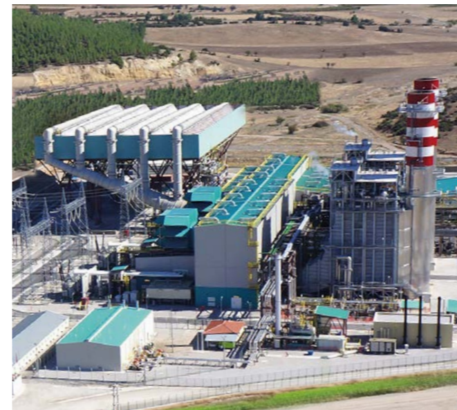
Combined Cycle Power Plant, Denizli Turn-key engineering, procurement and construction for a state-of-the-art natural gas fired combined cycle power plant, with a net power output of 775 MW . Turkey
