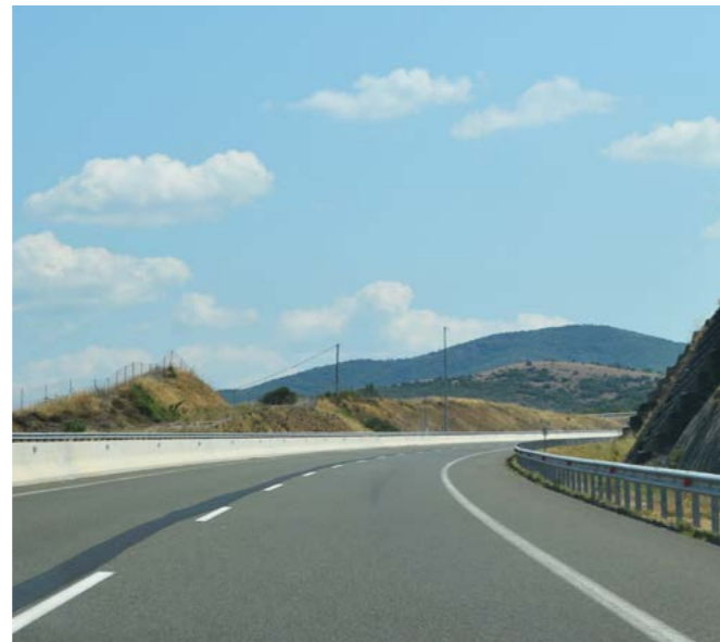
Aktio-Amvrakia Motorway Scope involves constructing 32 km of the new motorway connecting Aktio with Ionia Odos. Greece . Currently in progress.
