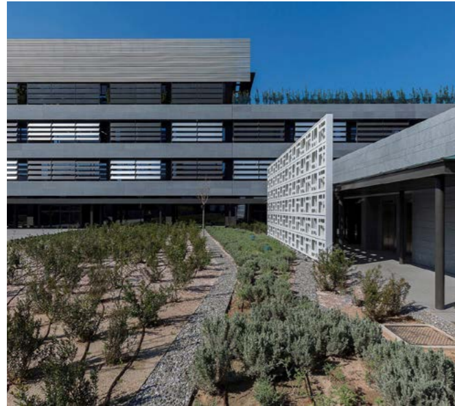
LEED Platinum Certified Building in Athens Construction of a multi-storey, 21,000 m 2 , LEED Platinum Certified Office Complex in Athens. Greece
