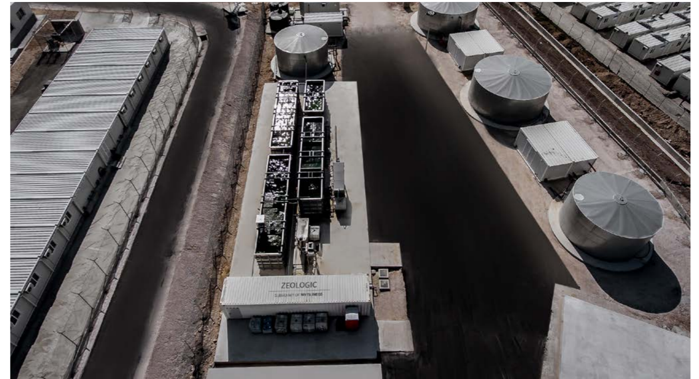
Liquid Waste and Potable Water Treatment Modularized Units with Zeologic technology. Greece
