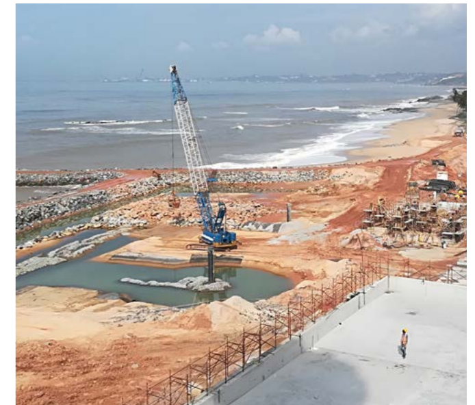
Amandi CCPP Marine Works Installation of one HDPE outfall pipeline DN280 of 350m, construction of a plumping wells system of 150m and construction of a 600m anti-scour protection in the sea front, using 50,000m 3 of stone material. Ghana
