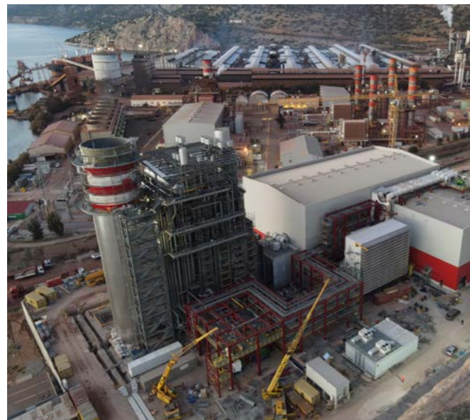
Ag. Nikolaos IPP II, Combined Cycle Power Plant Engineering, procurement, construction and commissioning of a 826 MW power plant in combined cycle (CCGT) configuration, operated by a GE H-Class gas turbine with a thermal efficiency of more than 63%, rendering the CCGT plant as the most efficient across Europe. Greece
