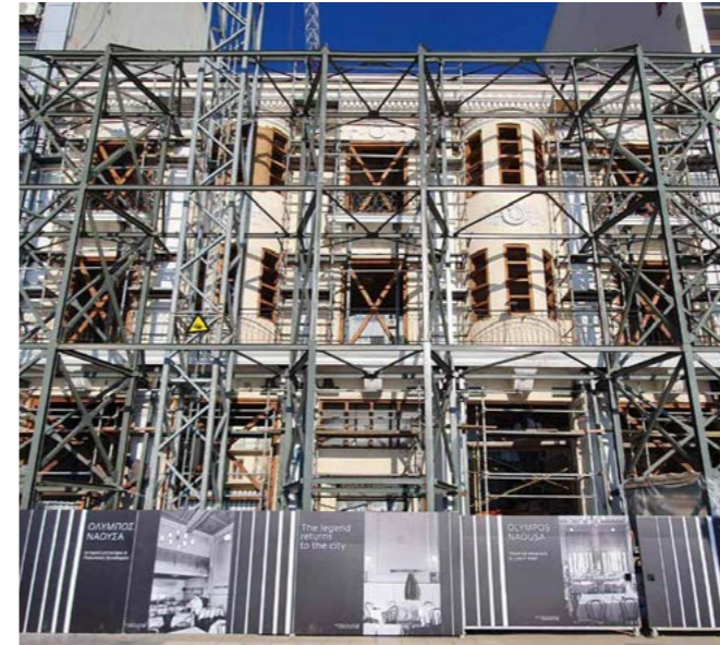
Olympos Naousa Hotel Renovation and extension of a historical and listed building, transforming it into a 5* Hotel, in Thessaloniki. Greece . Currently in progress.
