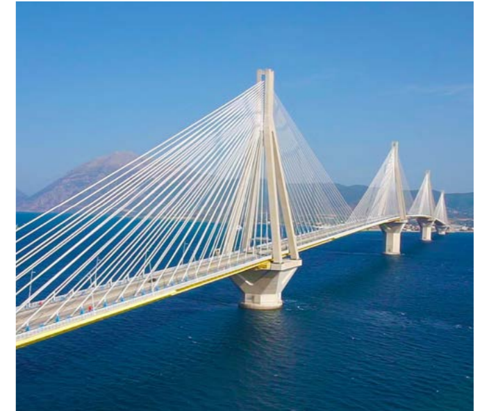
Rio-Antirrio Bridge Steel Works Scope involved the delivery of the head steel structures of the pylons of the impressive suspension Rion-Antirrio Bridge. Greece
