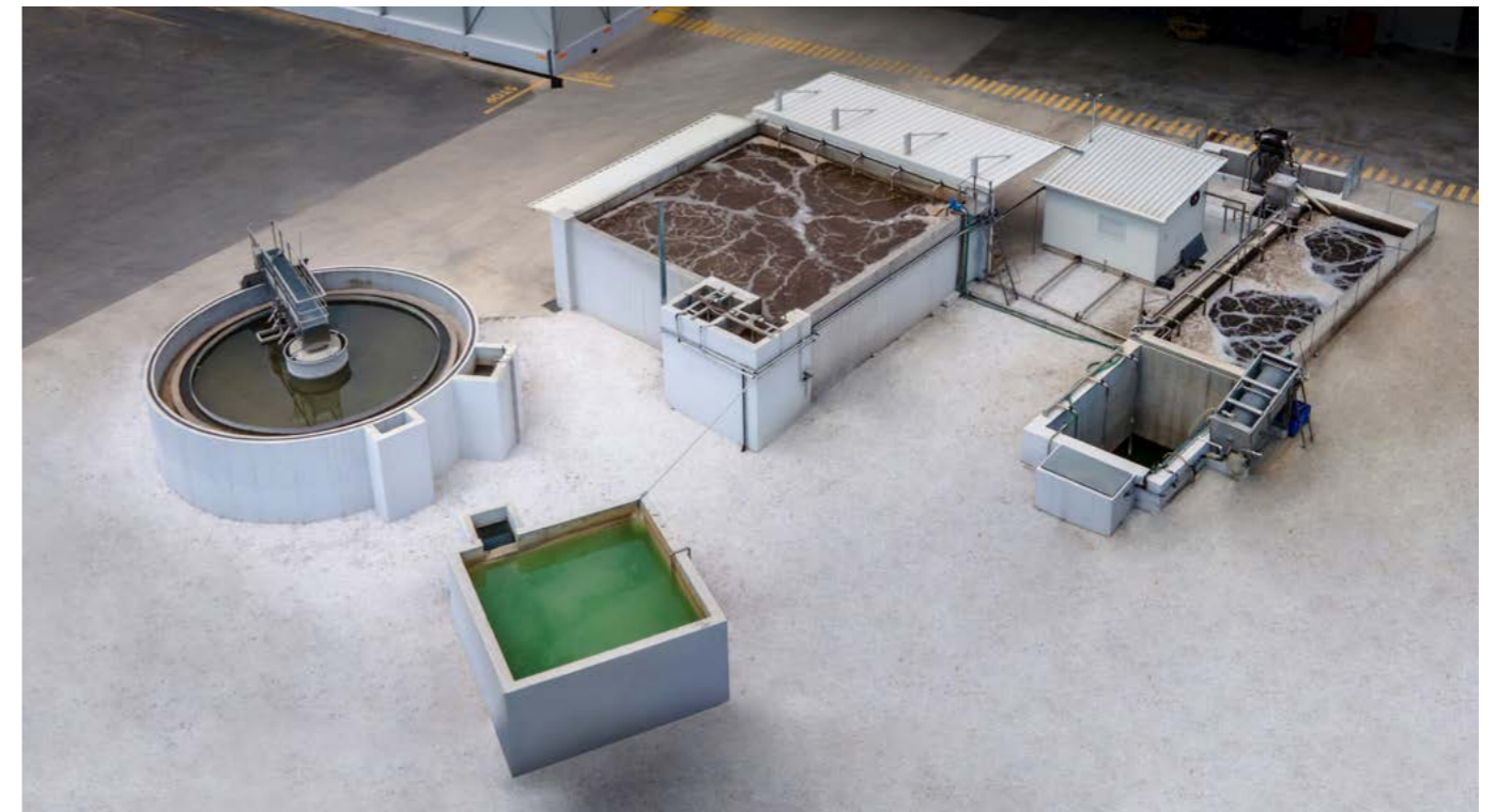
Wastewater Treatment Plant (WWTP) for the food processing industry (fruits and vegetables) with Zeologic technology. Greece
