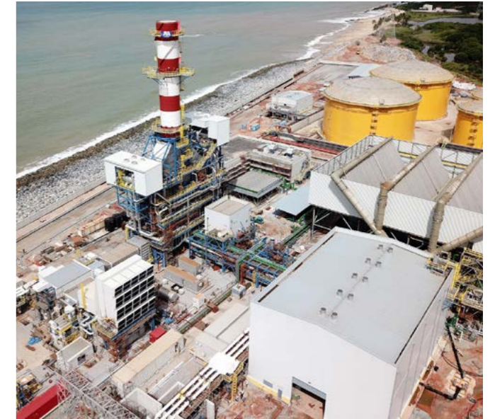
Combined Cycle Power Plant, Takoradi Engineering, procurement, construction and commissioning of a 192 MW , with the capability to operate on both natural gas and light crude oil. Ghana
