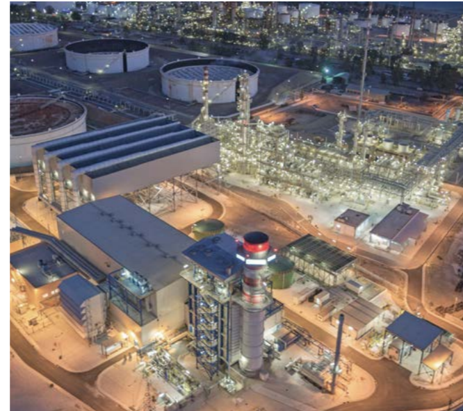
Korinthos Power S.A., Combined Cycle Plant Engineering, procurement, construction and commissioning of a 437 MW combined cycle gas turbine natural gas fired power plant. Greece
