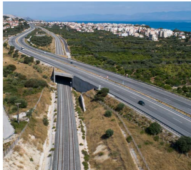
Kiato-Rododafni Railway Line Completion of a 71 km long new double-track high speed railway line, including signalling, telecommanding and telecommunications, from Kiato to Rododafni. Greece
