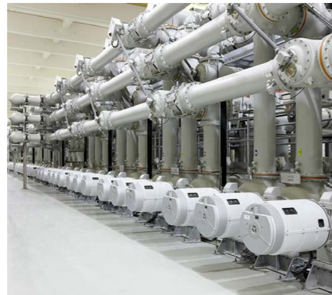
High-Voltage Substation (GIS) 400/150 KV, Aliveri Design, supply of equipment and installation of one high voltage gas insulated substation (GIS) of 400/150 KV . Greece
