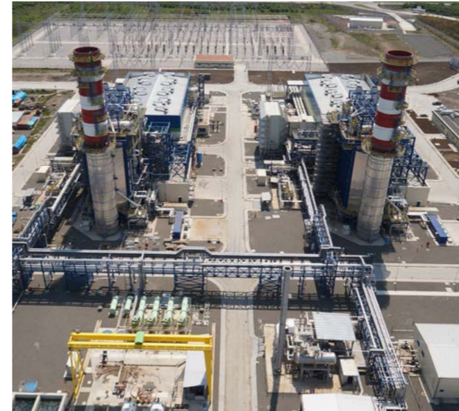
Combined Cycle Power Plant, Samsun Engineering, procurement and construction of a natural gas fired power plant, of 870 MW consisting of 2 combined cycle units. Turkey
