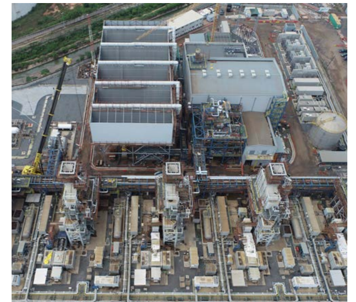
Power Plant of 200MW, Tema Engineering, procurement, construction and commissioning of a 200 MW power project in combined cycle (CCGT) configuration. Ghana
