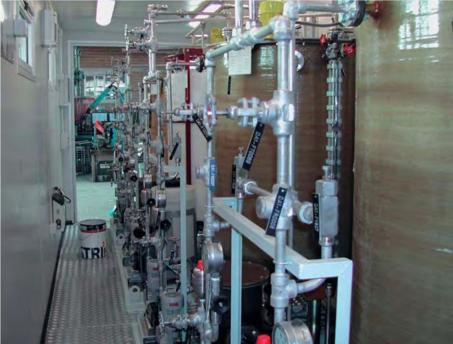
If one of the pumps of the dosing system breaks down, spare pumps will be manually or automatically activated.
