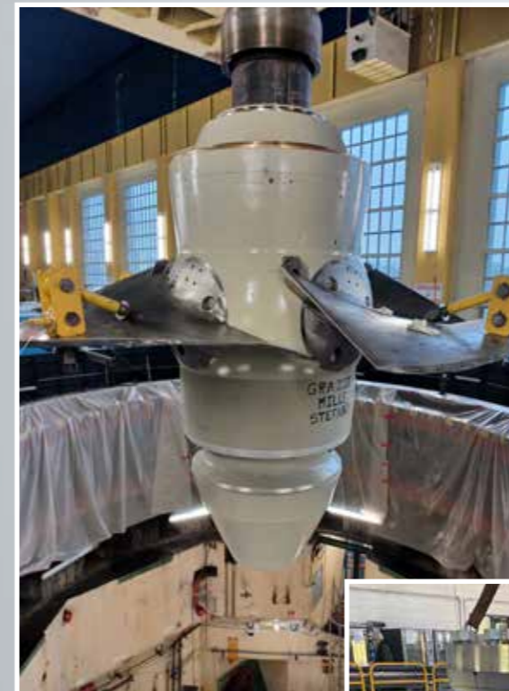
KAPLAN TURBINE INSTALLATION AT PLANT
