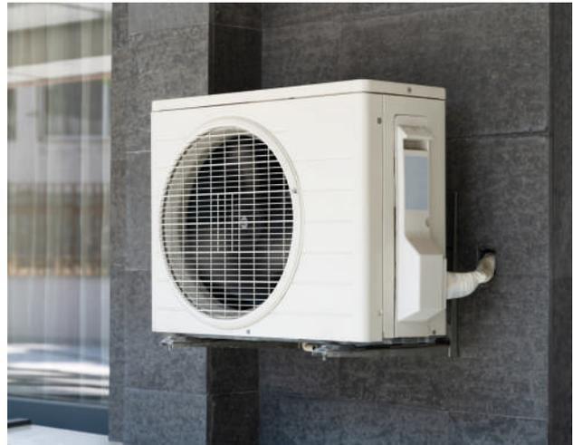
*On average, heat pumps for residential heating produce four times more thermal energy than they consume in electricity. They are a major lever for energy efficiency and for the decarbonization of heating.*
