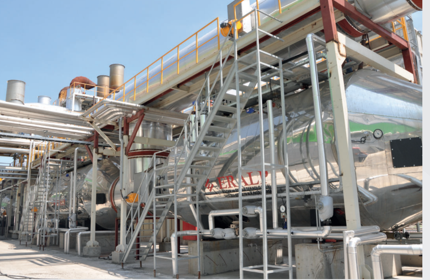
ALEV DUMAN BORULU ATIK ISI KAZANI FIRE TUBE WASTE HEAT RECOVERY BOILER
