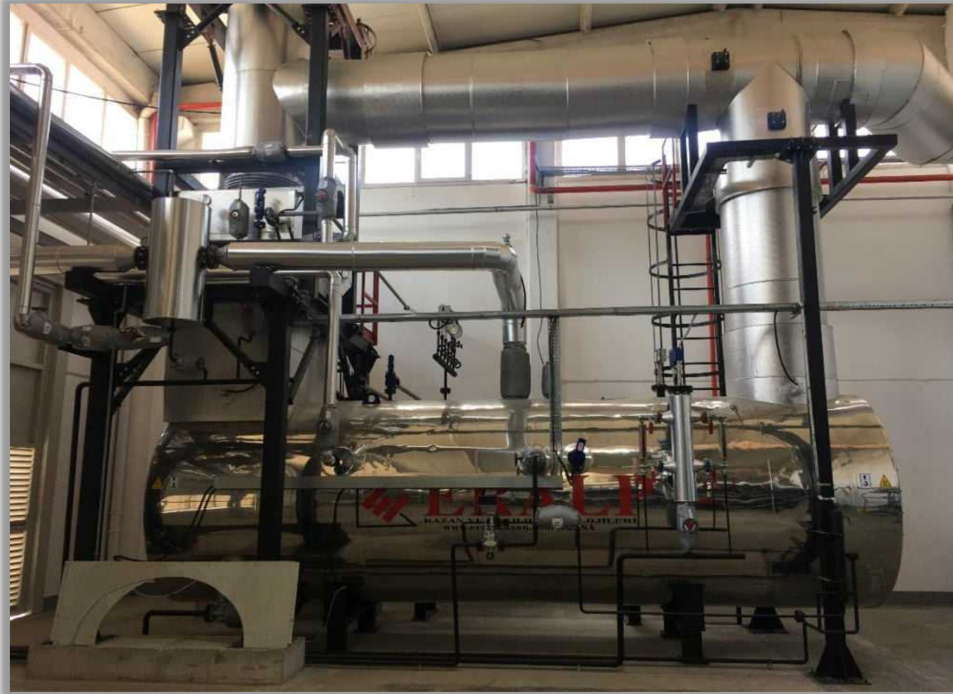
WHRB after 3 MW Gas Engine
