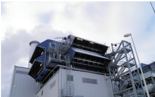
Filterhouse Upgrade from 2 to 3 Levels; Installation of EvapCooler for 2 Units F-Class
