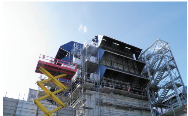
Filterhouse Upgrade from 2 to 3 Levels; Installation of EvapCooler for 2 Units F-Class
