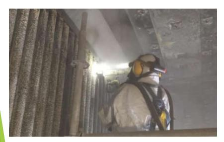
Cryogenic cleaning of HRSG tubes allows the removal of deposits that constitute an obstruction to the air/fume passage, resulting in a decrease in efficiency and an increase in Differential Back pressure
