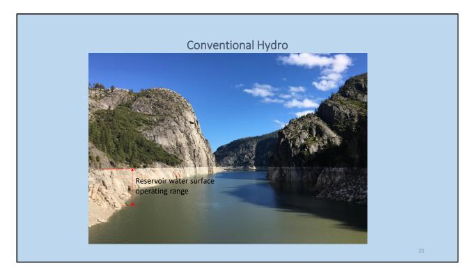
Donnells Reservoir normally operates within a 195 vertical foot range supporting Pelton turbines approximately 8 miles downstream operating under an average net head of 1,238 feet.
