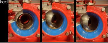
Gating down is used to change the flow through a line requiring less pressure than the master discharge pressure which is set for the highest line pressure required.
