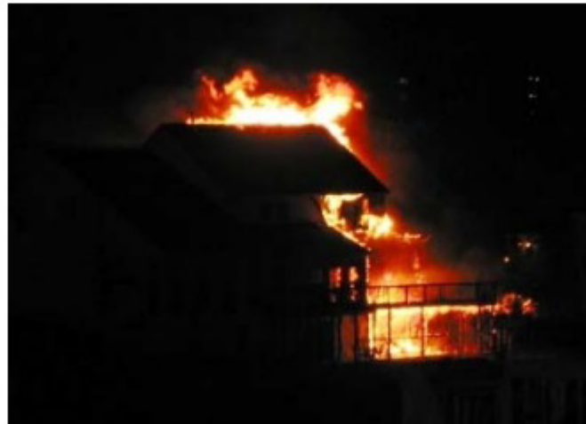
Side C view from neighbor's house Eiderdown Ct. prior to arrival of fire and rescue units
