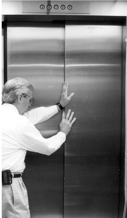
Fig. 1.3.4(c) Opening of Car Door by Hand (Not Possible on Some Elevators)
