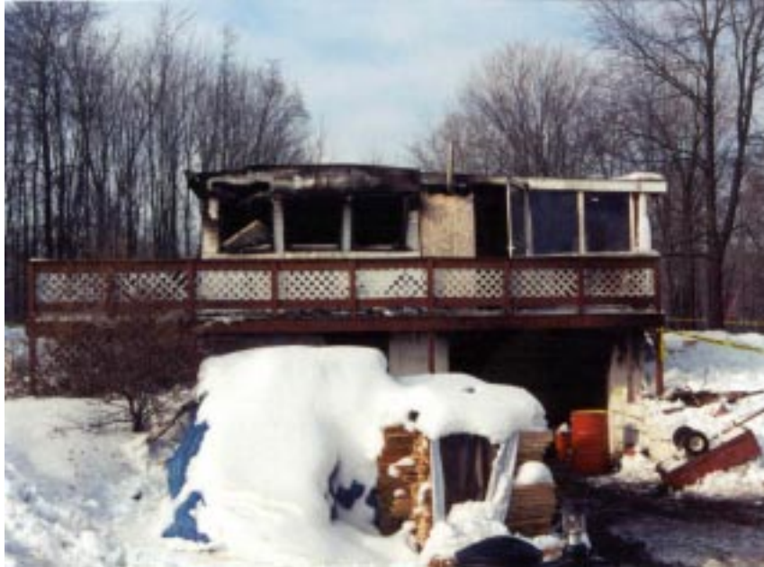
Photo 5. Entrance to Garage and Basement Area (Side 2)
