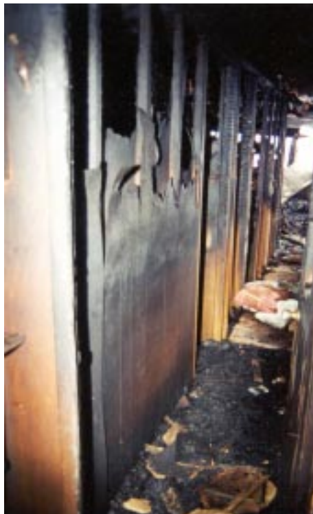
Photo 6. Hallway to Corner Bedroom
