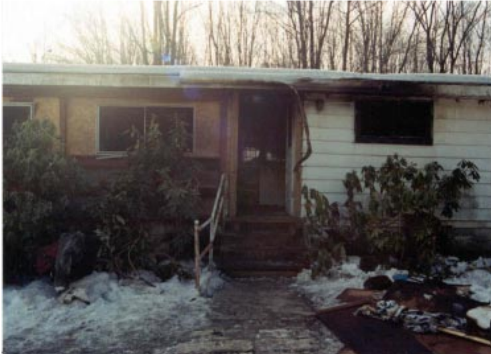
Photo 1. Front Door Entrance to Mobile Home (Side 1)
