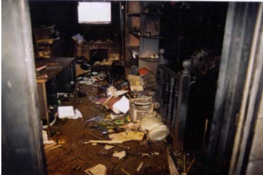
Photo 3. Addition to Mobile Home (12 ft x 12 ft)
