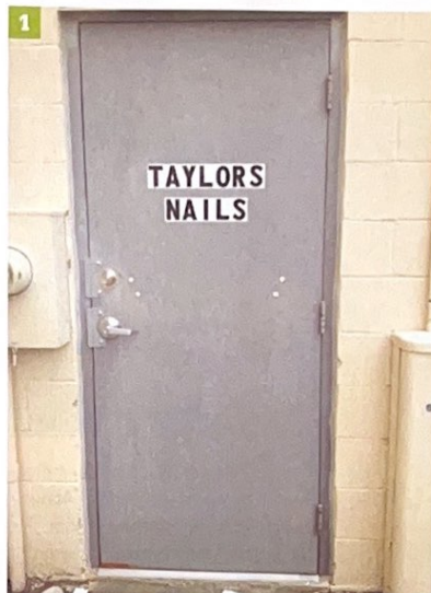
(1) Notice the carriage bolt pattern, key-in-knob lock with latch guard, and deadbolt. (Photos 1 and 3 courtesy of Rise Above Fire Training, LLC.) (2) One drop bar is present, in the middle of the door. The pull handle is indicative of panic hardware. (Photo by author.) (3) Notice the carriage bolt pattern, which is indicative of barrel bolts at the top and the bottom with a mortise lock.
