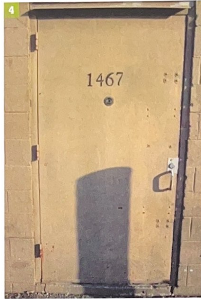
(4) Notice the presence of carriage bolts, indicative of multiple different locking devices such as barrel bolts. (Photos 4-5 courtesy of Rise Above Fire Training, LLC.) (5) The interior view of the door pictured in photo 4. Notice how the exterior size-up does not match what is found on the interior. This is proof positive of why we should always start with gap, set, force.
