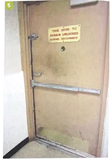
(4) Notice the presence of carriage bolts, indicative of multiple different locking devices such as barrel bolts. (Photos 4-5 courtesy of Rise Above Fire Training, LLC.) (5) The interior view of the door pictured in photo 4. Notice how the exterior size-up does not match what is found on the interior. This is proof positive of why we should always start with gap, set, force.
