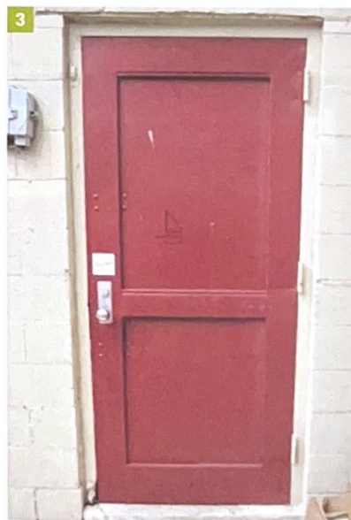
(1) Notice the carriage bolt pattern, key-in-knob lock with latch guard, and deadbolt. (Photos 1 and 3 courtesy of Rise Above Fire Training, LLC.) (2) One drop bar is present, in the middle of the door. The pull handle is indicative of panic hardware. (Photo by author.) (3) Notice the carriage bolt pattern, which is indicative of barrel bolts at the top and the bottom with a mortise lock.
