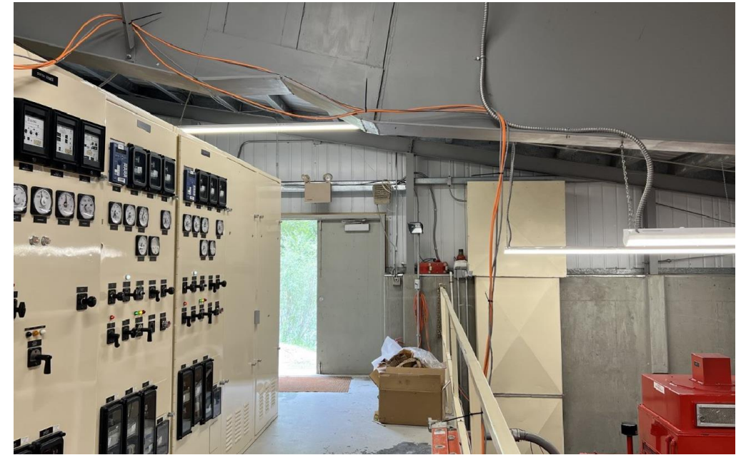
Cable retrofit for feedback and actuation
