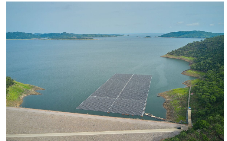
Bui Dam Ghana
