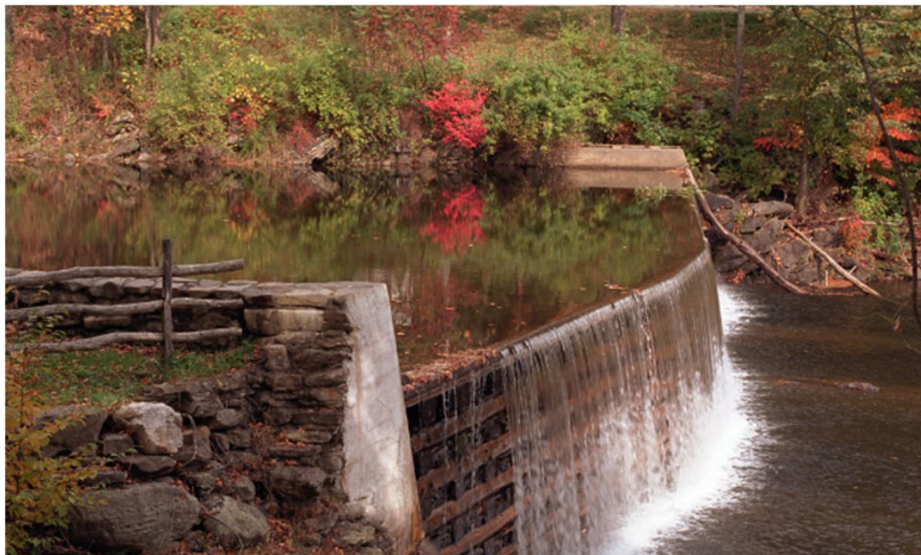
Timber Crib Dam
