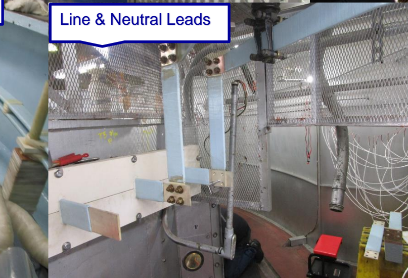
Pole Group Jumper Connections
