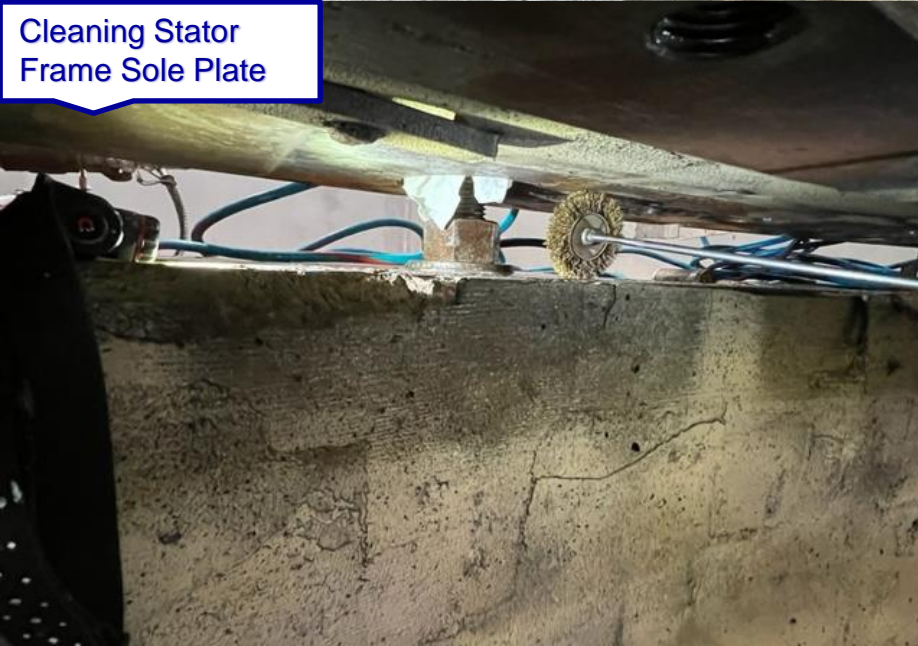
Stator Frame Sole Plate Cleaned and Lubricated
