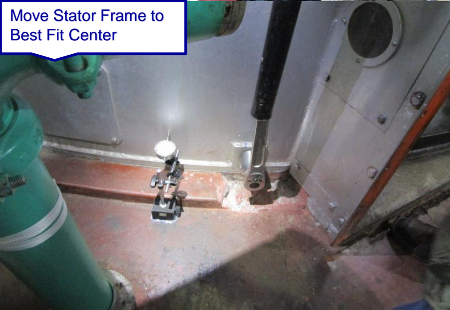
Stator Frame Laser Measurements Final
