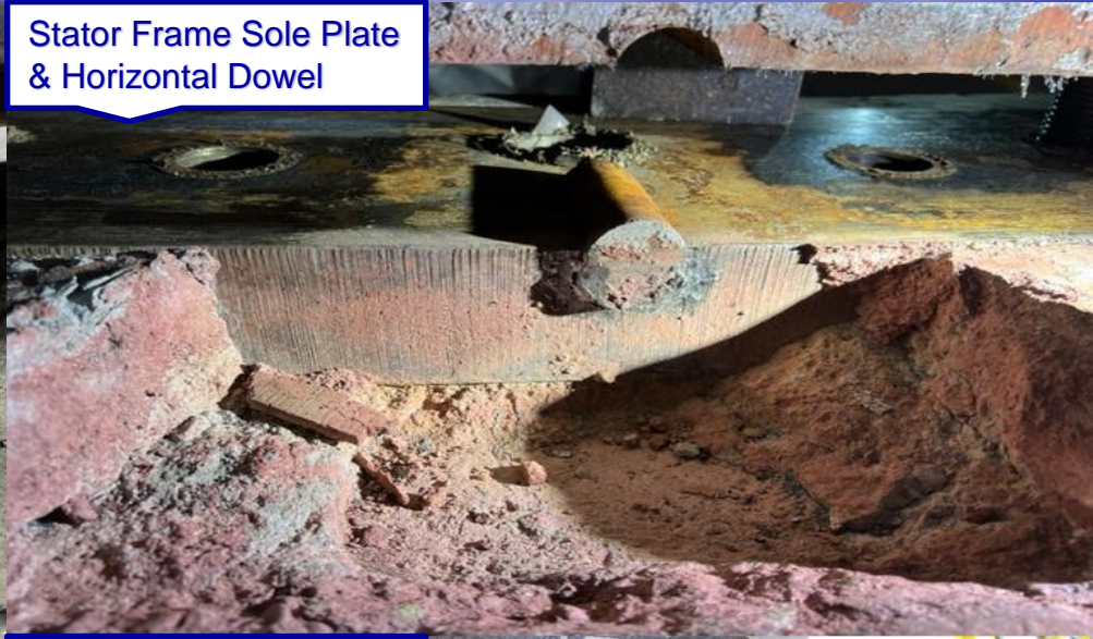
Stator Frame Sole Plate Cleaned and Lubricated
