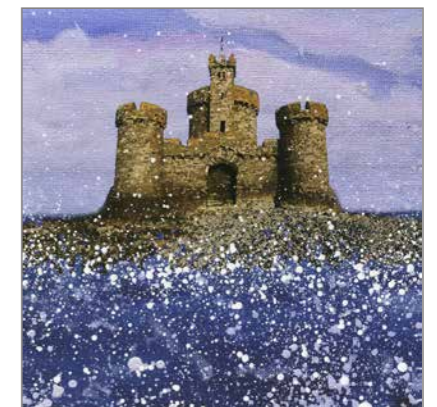
3IOM Tower of Refuge
