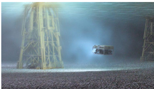
Fig. 8. ROVCO in the UK is applying SLAM with Machine Learning and specialist underwater imaging technology to vastly improve the fidelity of underwater asset inspection and intervention [8]
