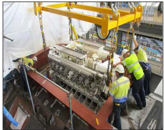
Fig. 3. Diesel engine being removed via a hull opening
