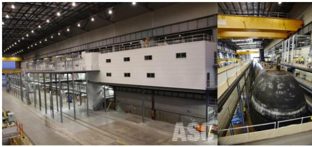
Fig. 2. Maintenance Support Tower in use during a Full Cycle Docking
