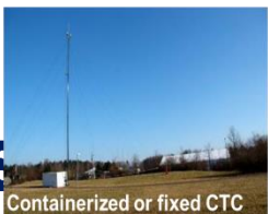
Containerized or fixed CTC
