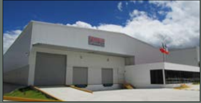
FERPER SPRINGS MEXICO PRODUCTION PLANT
