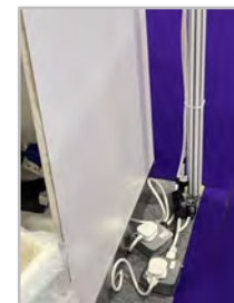
Socket attached to shell scheme wall pole Permitted
