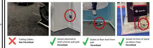
2. How To Position Power Sockets To The Front Of Shell Scheme Stand Space Without A 40mm Raised Floor
