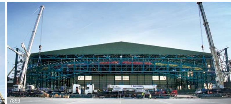
Above: Selection of REIDsteel hangars • Below: 140 tonne truss being lifted into position for a 100m span x 12m deep extension
