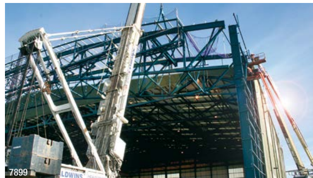
Above: Selection of REIDsteel hangars • Below: 140 tonne truss being lifted into position for a 100m span x 12m deep extension
