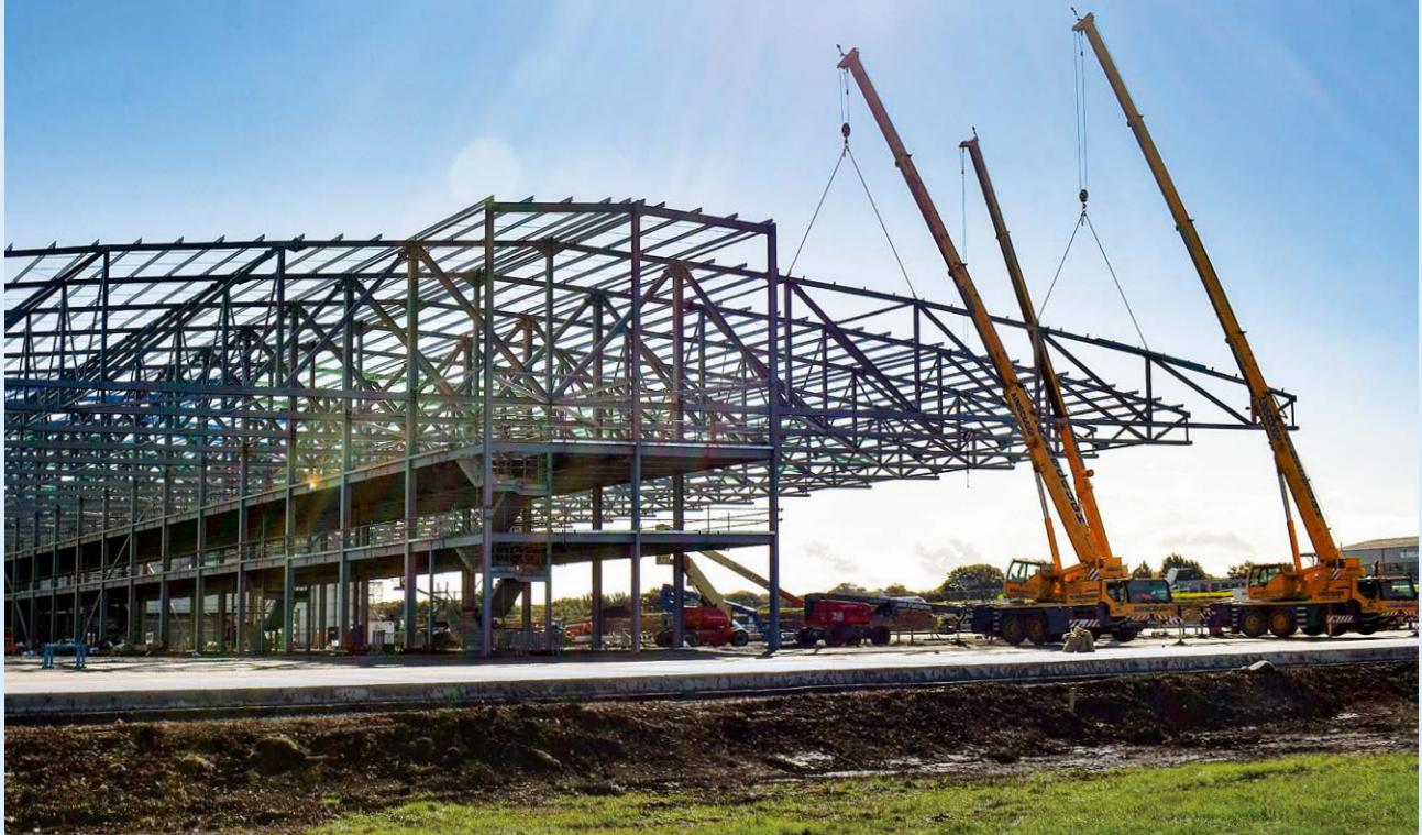
the deflection limits were extremely tight on this project due to the presence of the underslung crane and bottom rolling hangar doors.
