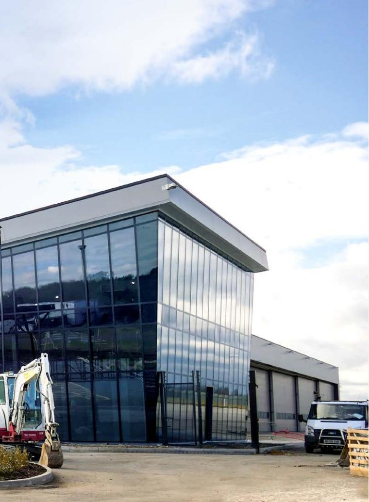
Early engagement of REIDsteel as the structural steel design and build fabricator, hangar door manufacturer and cladding was necessary given the need for elements to be erected and aligned on 45m cantilever trusses with requirements to accommodate complex hangar door head gear and underslung cranes – both of which required more stringent deflection criteria than usually anticipated on a large span structure.
