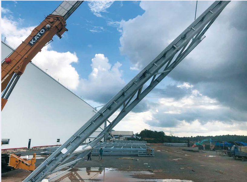
The hangar doors - hanging of the frames, cladding and finished.
