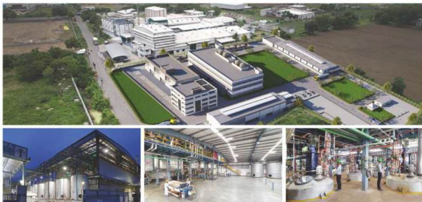
Manufacturing Facility- Rajsha Chemicals, Vadodara
