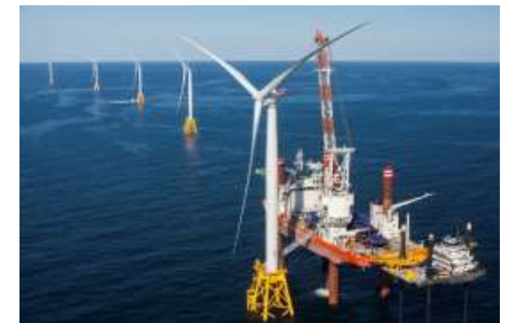
Heavy lift installation vessel
