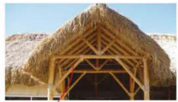
Bamboo and thatch shelter
